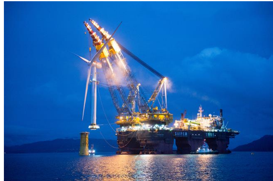
Deployment of offshore wind turbines that are going to supply the O&G platforms
